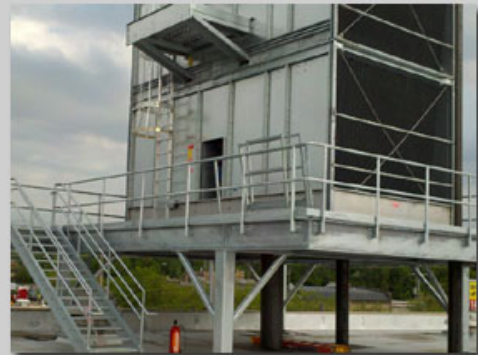
Exterior Cooling Tower
